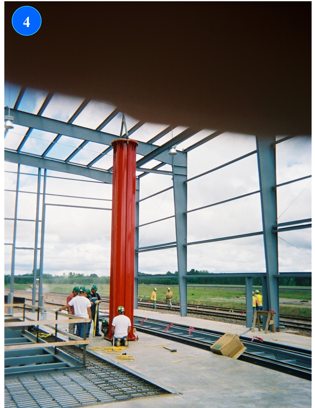
4 Bolt pedestal down to mounting pad and torque nuts.
