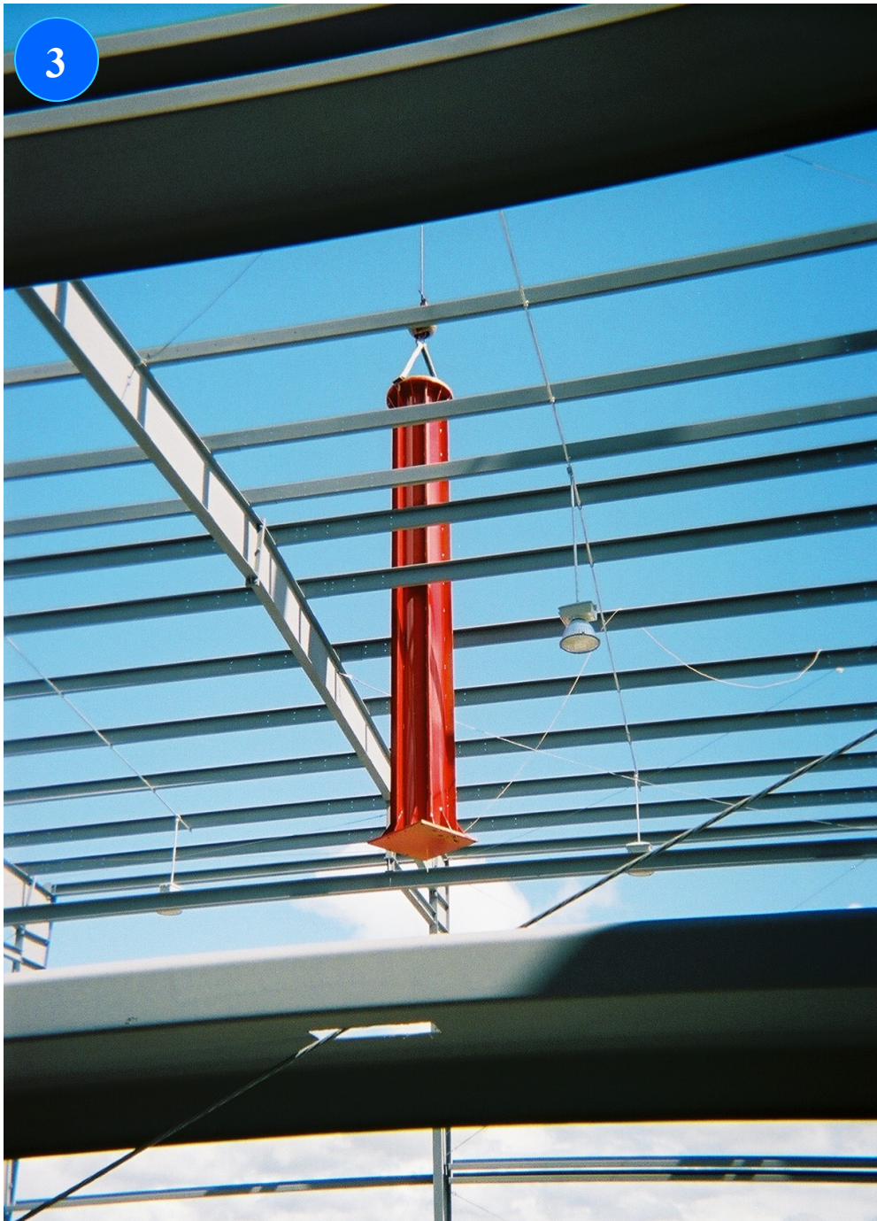
3 Lower pedestal into place.
